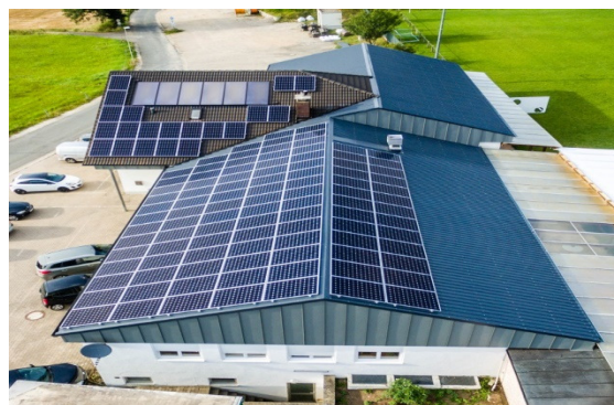
39 kWp DJK Weingarts
